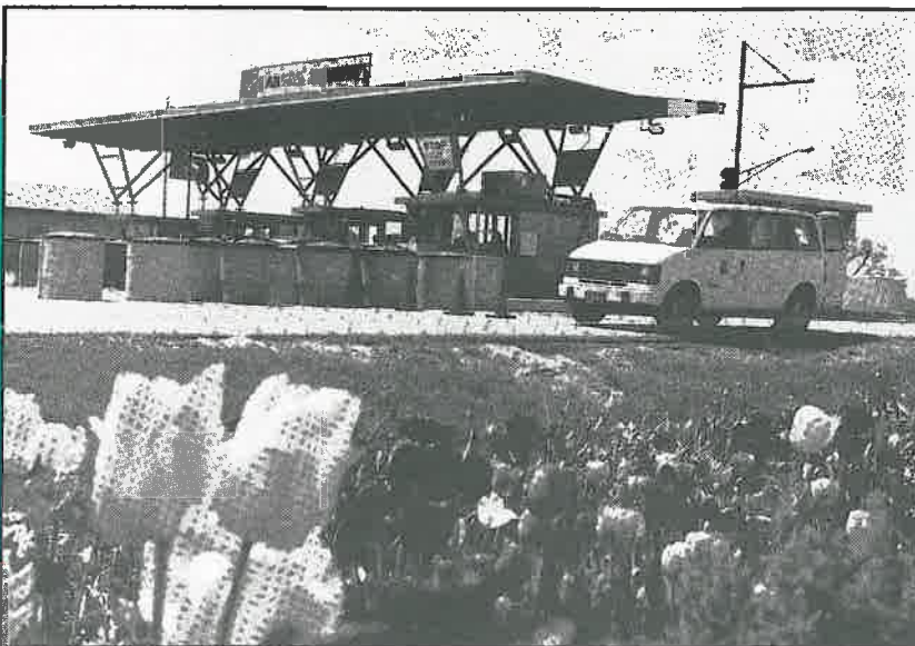
Colorful tulips bring signs of spring and welcome motorists to this Kansas Turnpike toll plaza. (Photo courtesy of the Kansas Turnpike Authority)
